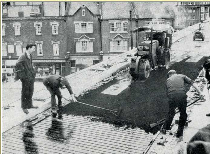
1969 Laying asphalt on the upper carriageway of a Hammerschmidt junction in London (Electric heating of the roadways, by Robert Félix, 1971, Ultimheat Museum* )
